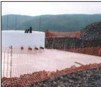
Foundations for wind turbines can be many feet deep and wide. A staggering amount of steel and concrete go into them.
