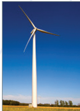
Large scale wind turbine
