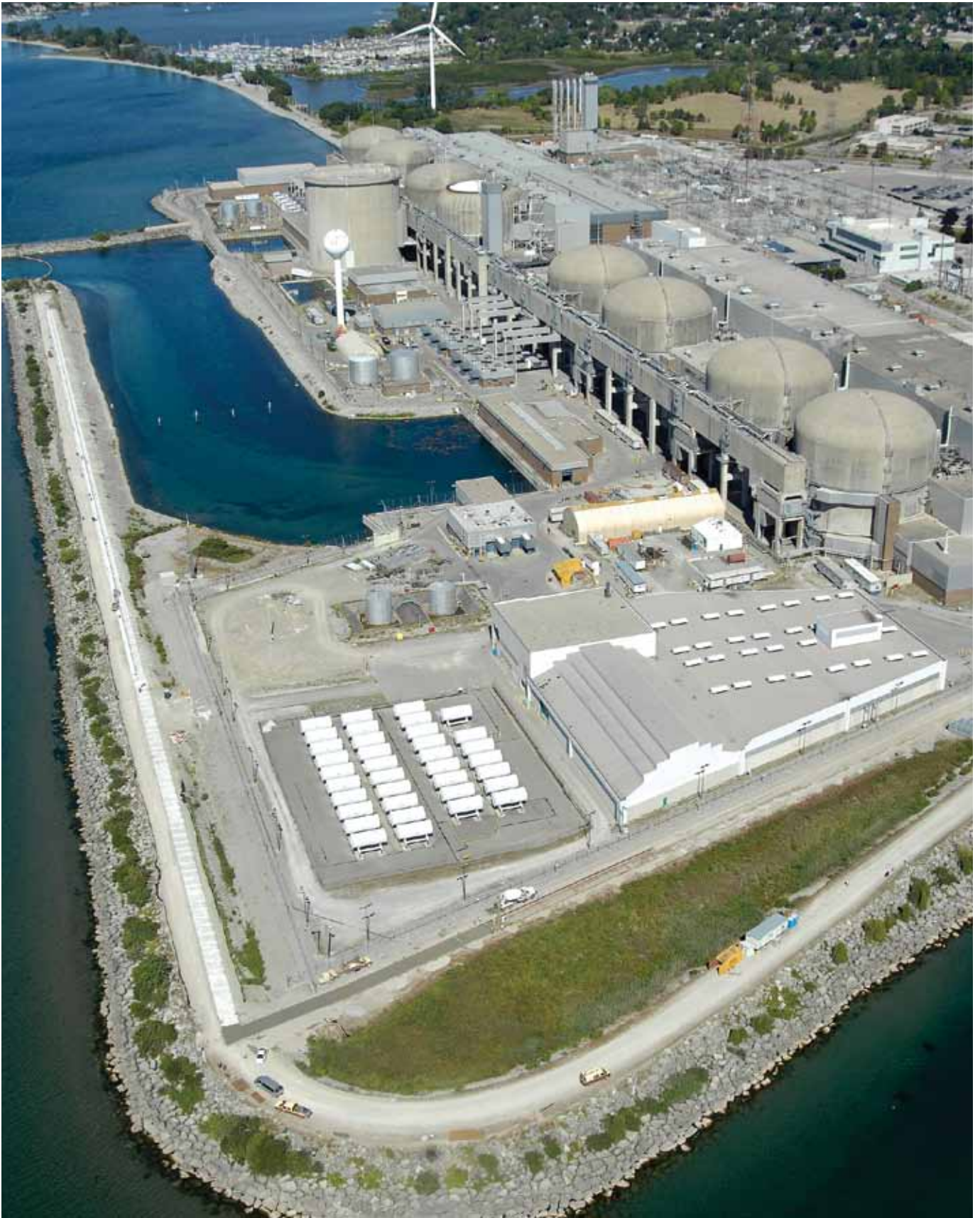
Photo: Courtesy Ontario Power Generation
