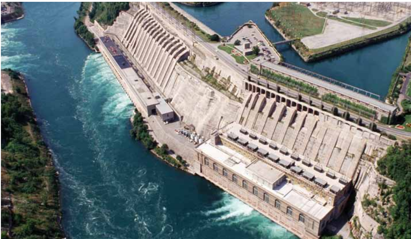
The Sir Adam Beck Generating Station at Niagara Falls: Ontario's best hydroelectric sites, including this enormous facility, have already been developed
